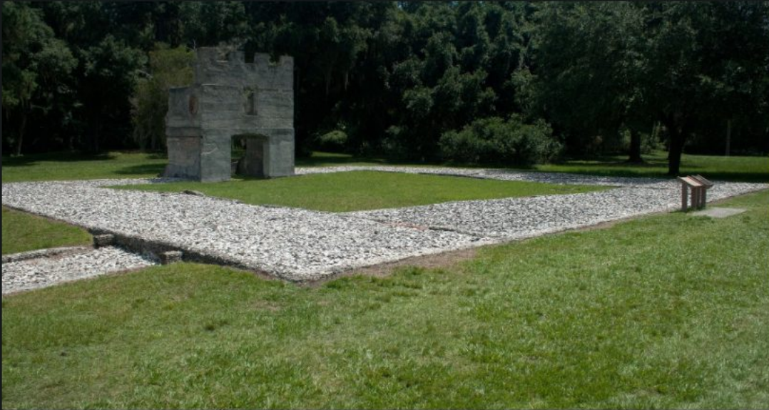
1736 Fort Frederica barracks. Tabby: oyster shell, lime, sand and water, poured in lifts.
